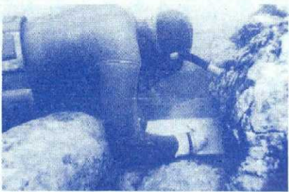
A diver measures concrete forms left behind from barrels of cement carried as cargo on the Edinburgh Castle.
